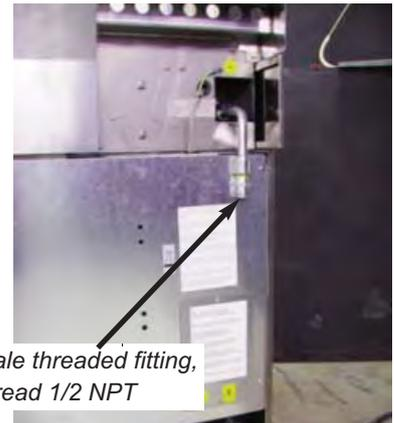
Install a manual gas line shut-off valve in the gas line in an easily accessed location outside of the range. Make sure everyone operating the range knows where and how to shut off the gas supply to the range.
