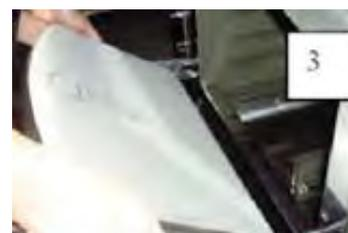
3. Remove the plinthes/toe-kicks using a standard screwdriver.
