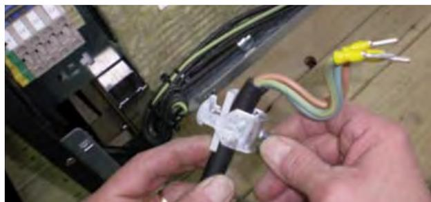
4. Insert the strain relief device into the hole and push it to the left. Tight up the power cord and strain relief device with the screw.
